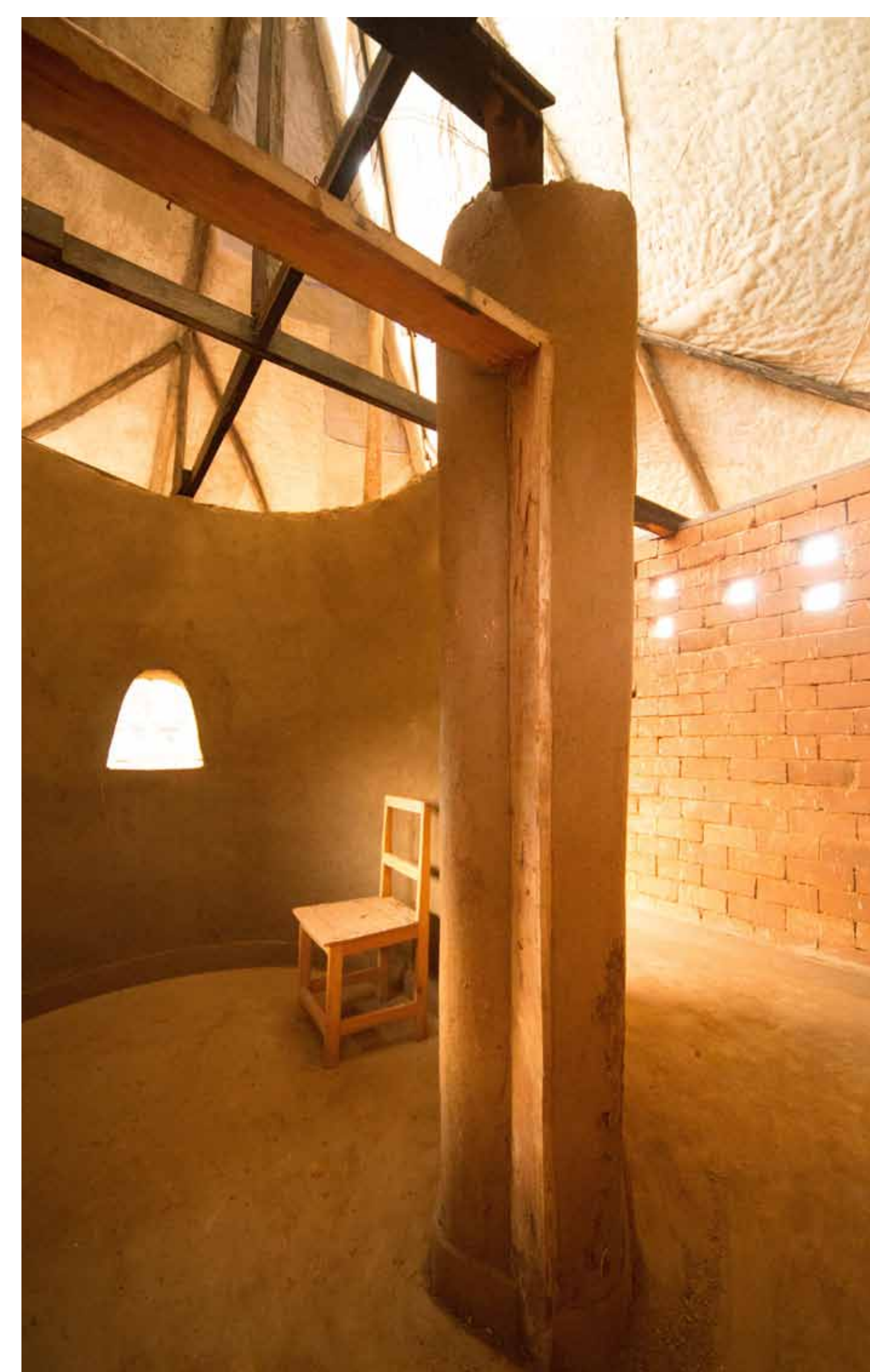
Experimental house, built by students of UR (Rwanda)
