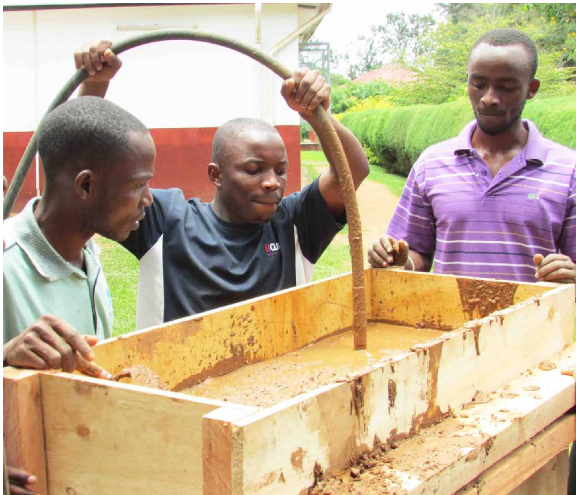
Experimental clay wall construction with students of UMU, Nkozi (Uganda)
