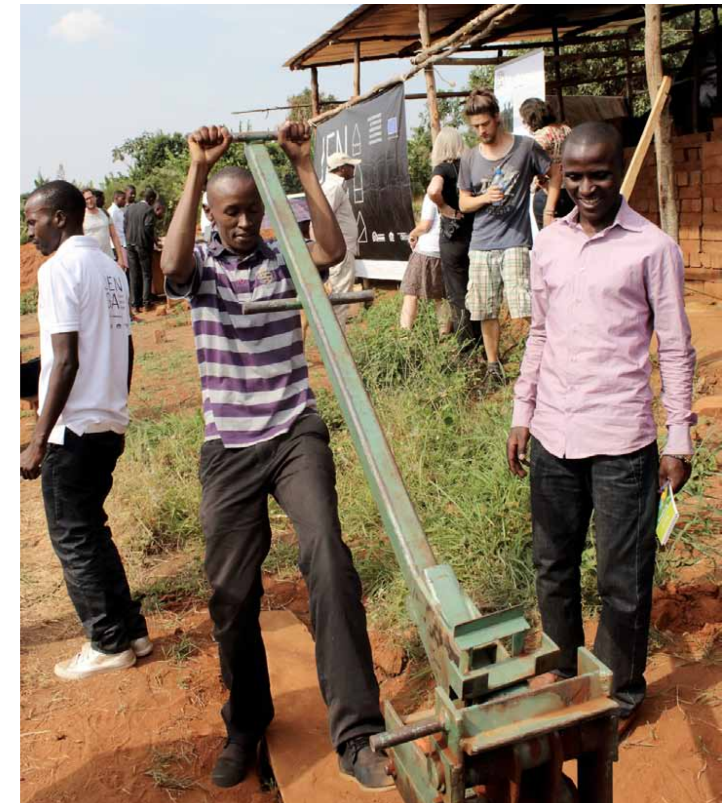
Stakeholders making clay bricks at UR design-build construction site, Rwinkwavu (Rwanda)
