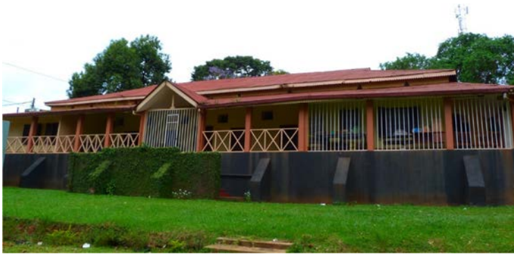
Figure 4: Kweerimidde House in 2017. (Source: Author, 2017.)
