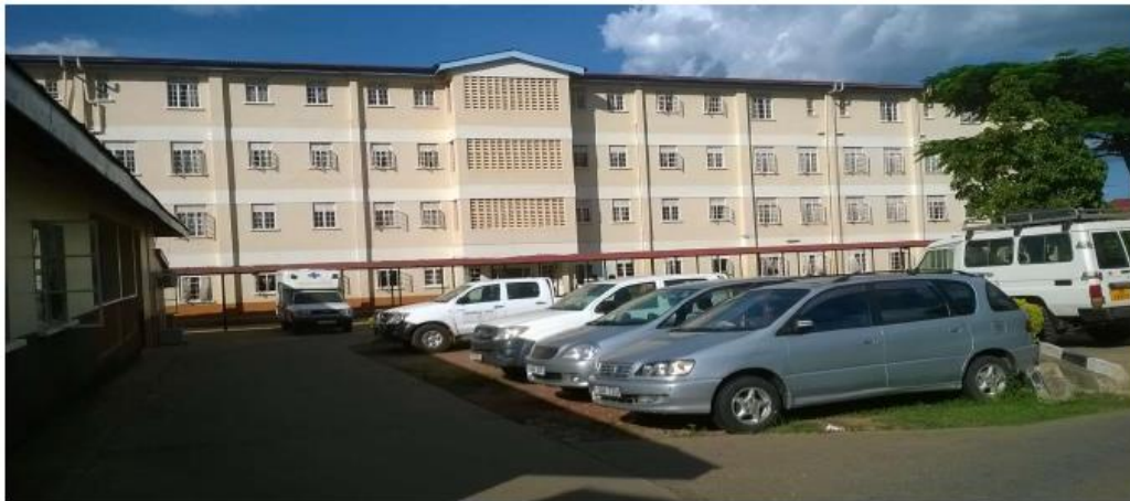
Figure 3. Arua regional referral hospital _ uganda
